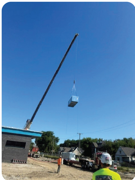
Booming up 5,000 lb. equipment
