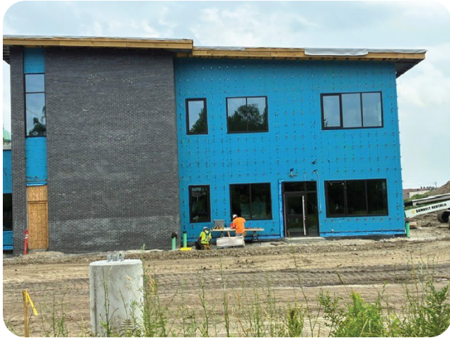
Exterior siding install starting
