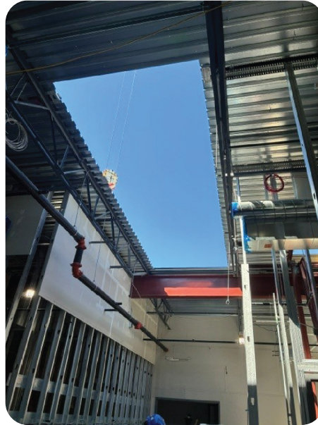
A hole was cut through roof for HVAC equipment delivery
